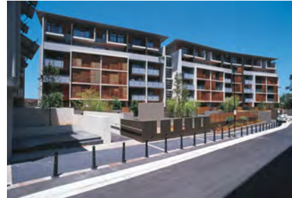
This facade has a strong balance of horizontal and vertical framing elements with sunscreen and balustrade infill components
