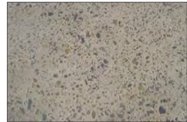
Insitu exposed aggregate concrete
