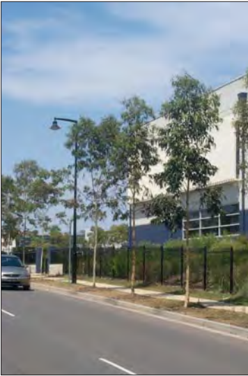
Concrete kerb and gutter
