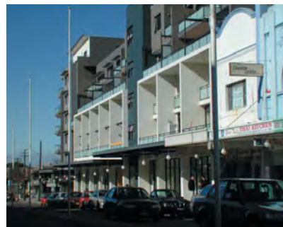
Variation in height of different floors adds to the articulation/visual quality of the building.
