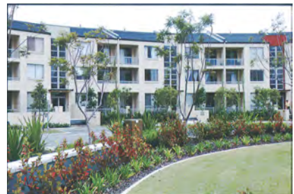
The use of multiple lift and stair cores promotes more entries along the street and can help to 'break up' a long building facade.
