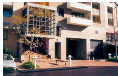
This elevation treats the car park entry as part of the whole elevation. It narrows the width of the entry and defines an opening in proportion to the other facade elements.
