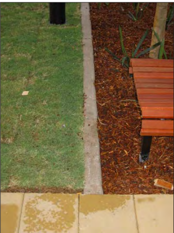
Concrete flush edge - exposed aggregate
