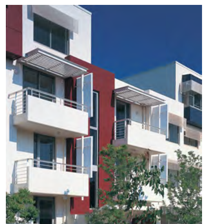
The detailed design of these partially solid balustrades, sun shades and privacy screens contribute to the overall facade composition of the building.
