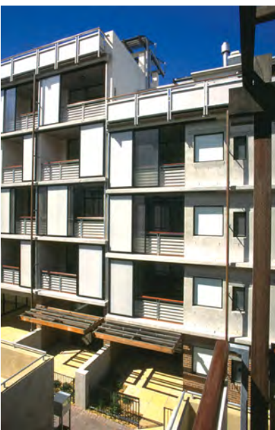
Building elements provide privacy between spaces, pergolas limit overlooking, solid walls and sliding screens limit horizontal views.
