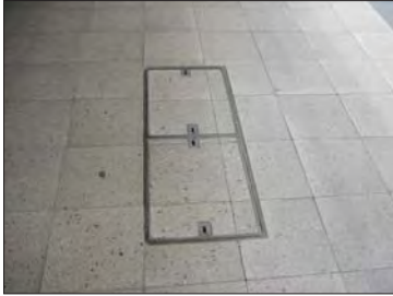
Paving infill lid in unit pavement
