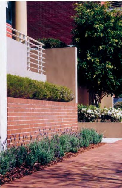
Materials and planting are combined in a good ratio of solid to void, to enhance visual amenity of the street, whilst ensuring privacy and security to the residents.
