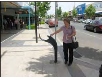
Exposed aggregate unit concrete pavement
