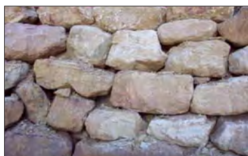
Sea wall edges should optimise the incorporation of niches and ledges that can enhance aquatic habitat
