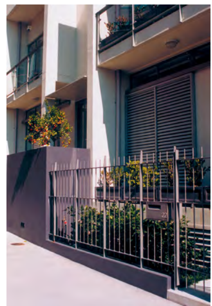
Street level picket fencing with planting provides screening to car park
