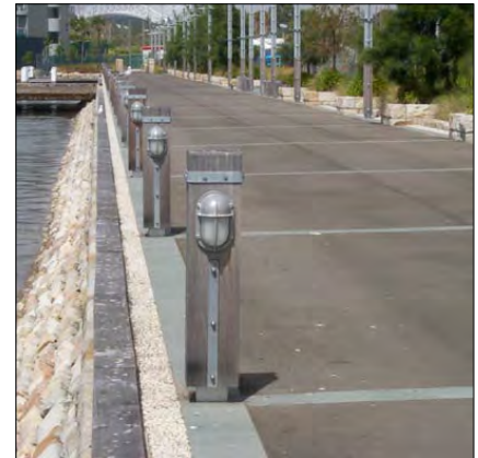
Existing asphalt pavement with granite banding adjoining PAYCE development
