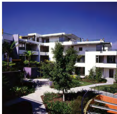
The site's topography has been used to create a series of smaller more intimate spaces using retaining walls and planter beds, which step down across the site.
