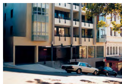
On this small site on a steep terrain, the entry and exit driveways are split to maintain a consistent scale of facade openings.
