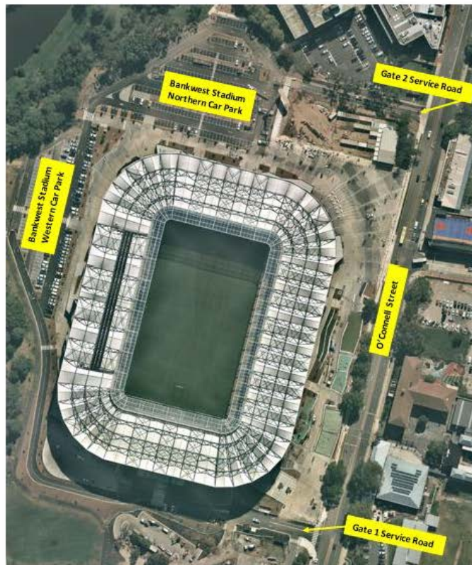
BANKWEST STADIUM – WESTERN AND NORTHERN CAR PARKS
