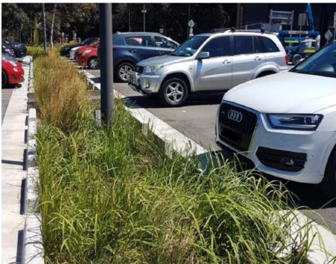
Swales in carpark or near other large areas of pavement collect stormwater runoff and remove pollutants
