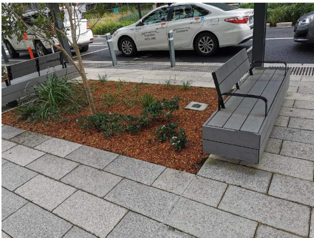
WSUD at Northern Beaches Hospital
