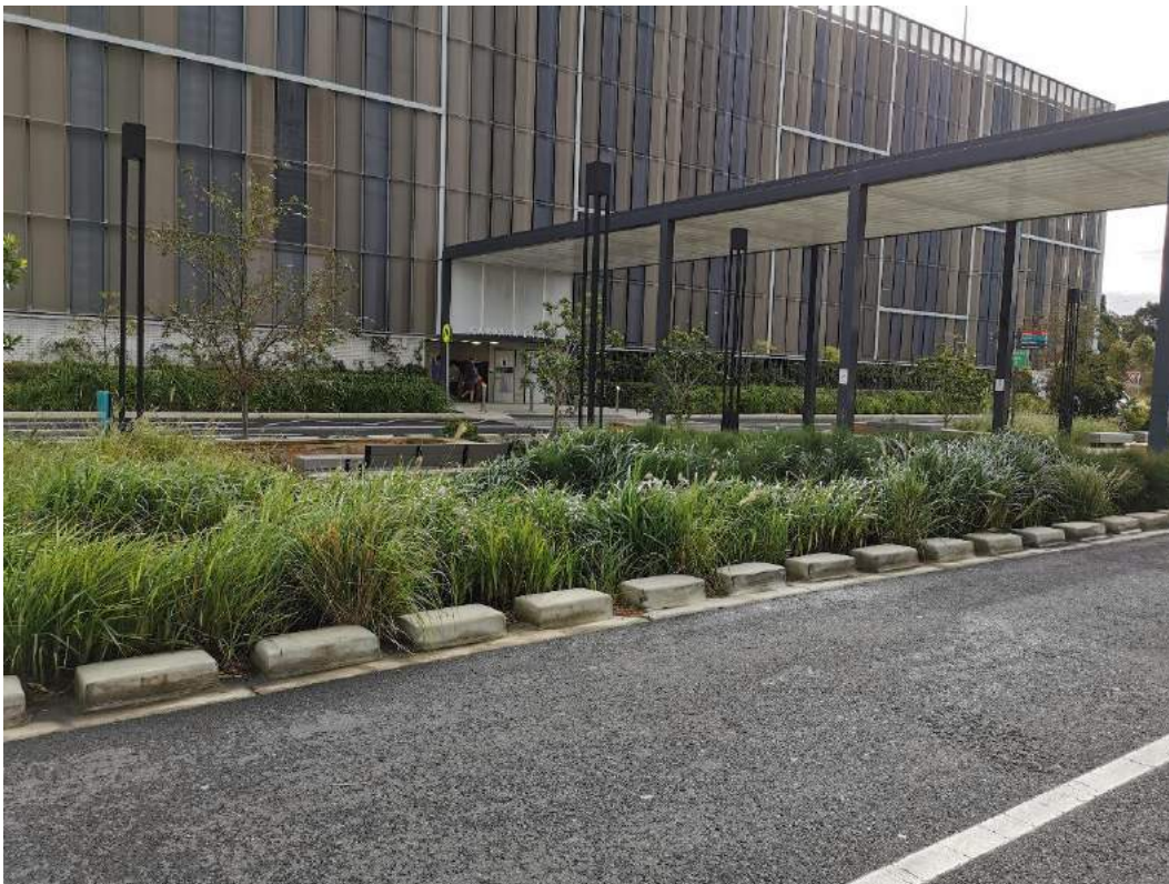
WSUD at Northern Beaches Hospital
