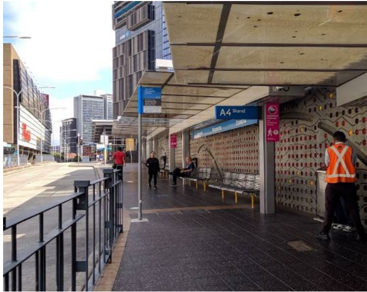
PTA11,12,13 Parramatta Stn-Bus Stop Stand B4
