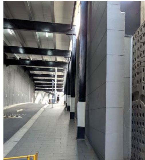
PTA56 Parramatta Stn-CCTV Cameras
