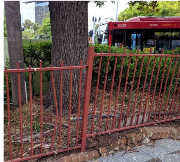
PTA50 Parramatta Stn-Walkway No1
