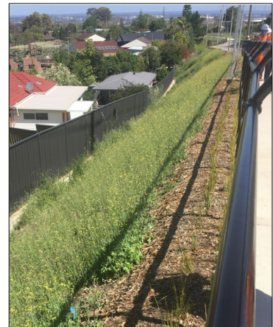
Figures 12A & 12B Examples of adverse effects of spoil retention – unsafe, difficult to maintain steep embankments and overlooking
