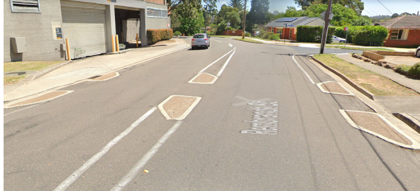
Figure 2: Street view of the non-compliant pedestrian island on Rembrandt Street south of Milton Street, Carlingford
