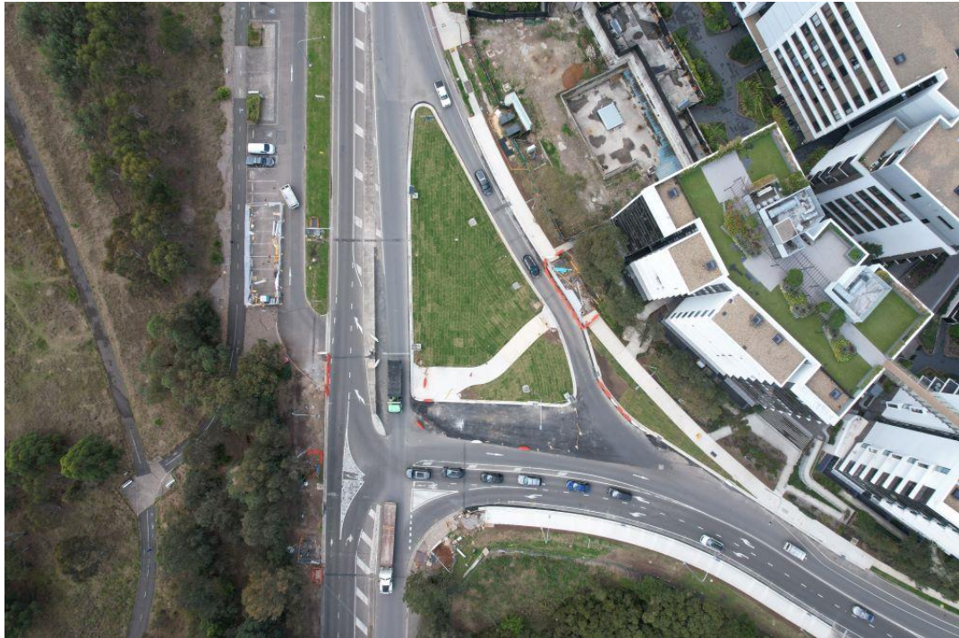
Figure 1: A drone captured image of the completed works at the intersection of Hill Road and Burroway Road, Wentworth Point
