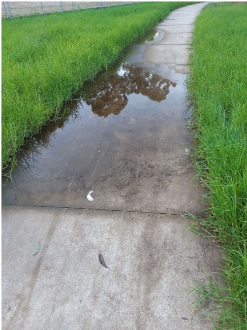
Figure 5 - Image showing pooling on pathway
