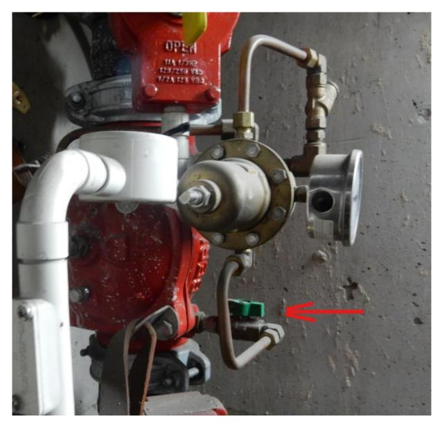
Appendix 3 - Image Pilot Operated Valve and Isolation Valves
