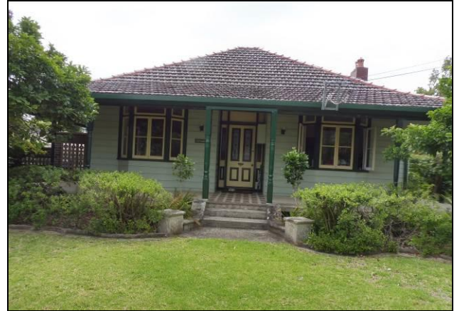
Figure 5.4 The front facade is symmetrical about a recessed entry and has an open, wrap around verandah. The verandah floor and details have been previously modified.
