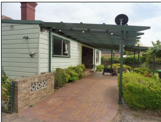
Figure 5.8 The rear wing retains the kitchen chimney and has a central, recessed verandah. A brick paved patio and timber pergola have been added to the rear. Removal of these elements has been approved.
