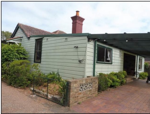
Figure 5.7 The rear skillion roof and south eastern corner of the building which has been extended and modified. Removal of the chimney and part of the rear wing has been approved.
