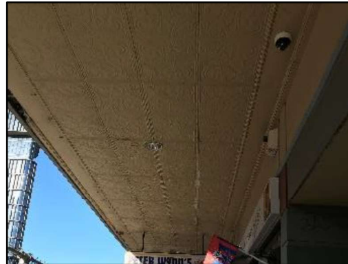
Figure 4. External view of the cantilevered awning showing the pressed metal ceiling of the Federation department store as viewed along Church Street.
