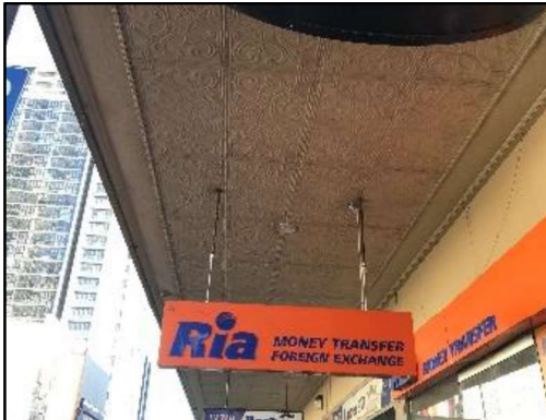
Figure 3. External view of the cantilevered awning showing the pressed metal ceiling of the Federation department store as viewed along Macquarie Street.
