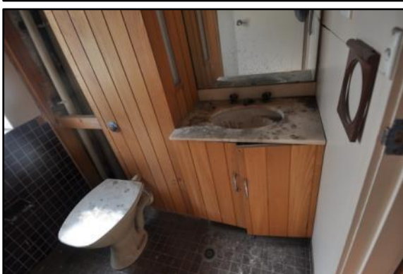
Figures 69, 70, 71 & 72: Kitchenette/bathroom areas at north-east corner. Fixtures and finishes are not original. Most surfaces in poor condition and damaged. Timber flooring and masonry wall visible.
