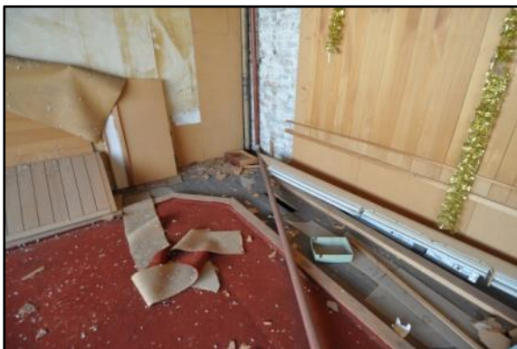
Figures 61, 62, 63 & 64: Main room on south side. Linings are not original and are peeling away. Most surfaces in poor condition and damaged. Timber flooring and masonry wall visible.
