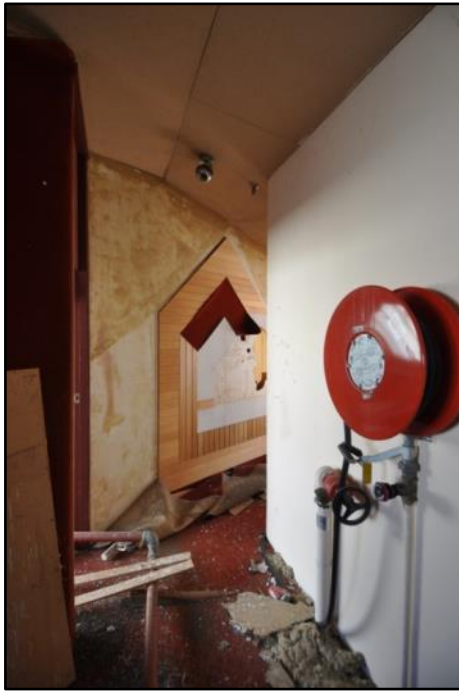
Figures 59 & 60: Central corridor. Linings are not original and are peeling away. Most surfaces in poor condition and damaged.
