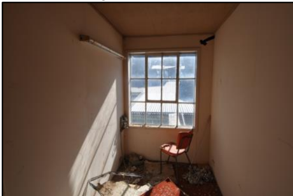
Figures 67 & 68: Room on north (left) and corridor where former staircase was. Linings are not original and are peeling away. Most surfaces in poor condition and damaged. Services have been inserted into the space.
