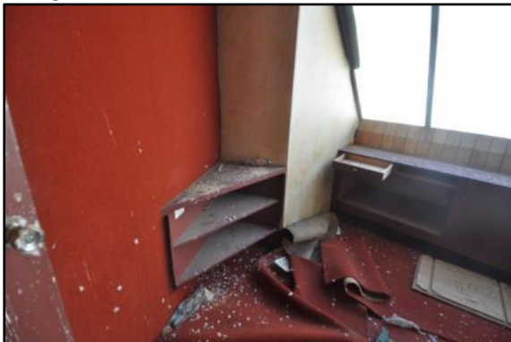
Figures 59 & 60: Central corridor. Linings are not original and are peeling away. Most surfaces in poor condition and damaged.
