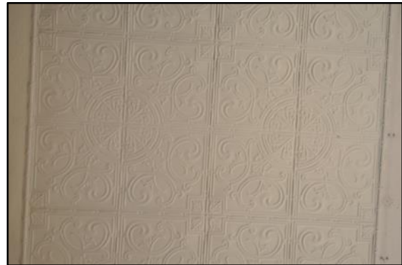
Figure 30: Detail of pressed metal undersides of awnings.
