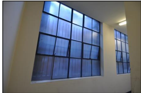
Figure 45: Steel windows in service corridor at rear of building. Contemporary wall, floor and ceiling finishes.
