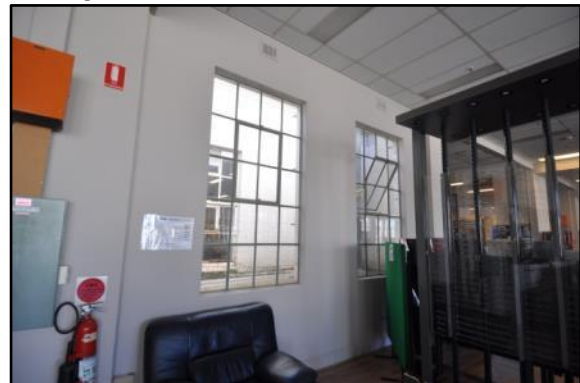
Figure 51: Interior with contemporary wall, floor and ceiling finishes. Original steel windows to lightwell.
