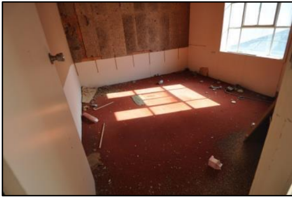
Figures 65 & 66: Interior of room at north-west corner. Linings are not original and are peeling away. Most surfaces in poor condition and damaged.
