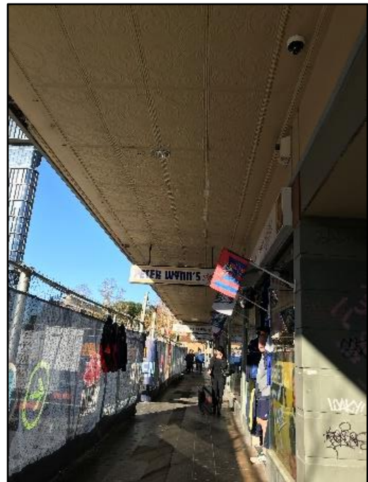
Figure 35. External view of the cantilevered awning showing the pressed metal ceiling of the Federation department store as viewed along Church Street.
