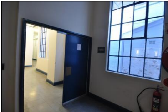
Figure 44: Service corridor at rear of building. Contemporary wall, floor and ceiling finishes. Original steel windows.
