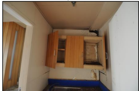
Figures 67 & 68: Room on north (left) and corridor where former staircase was. Linings are not original and are peeling away. Most surfaces in poor condition and damaged. Services have been inserted into the space.
