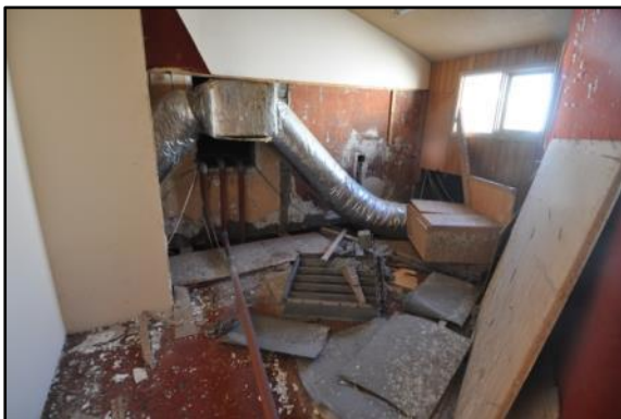
Figures 57 & 58: South-east corner. Services have been inserted into the space. Linings are not original and are peeling away. Most surfaces in poor condition and damaged.
