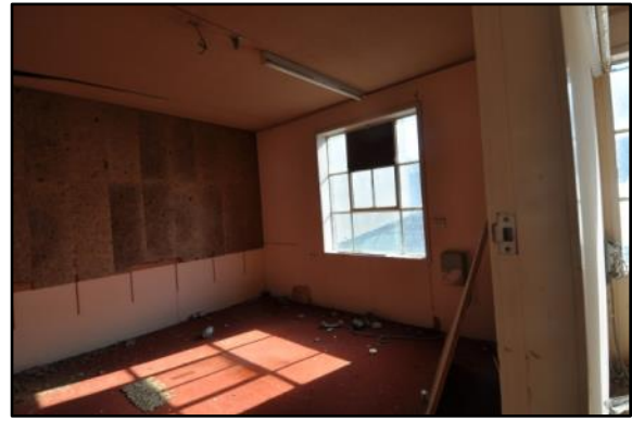
Figures 65 & 66: Interior of room at north-west corner. Linings are not original and are peeling away. Most surfaces in poor condition and damaged.
