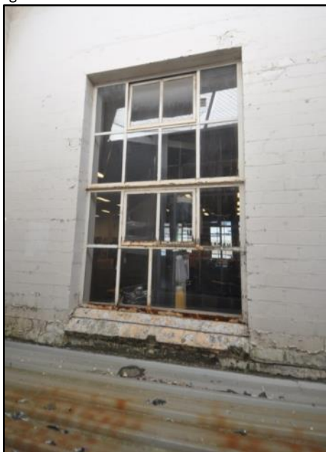
Figure 52: Detail of steel windows to light well showing hopper style openings and corrosion.
