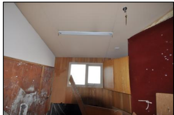
Figures 57 & 58: South-east corner. Services have been inserted into the space. Linings are not original and are peeling away. Most surfaces in poor condition and damaged.
