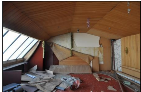
Figures 59 & 60: Central corridor. Linings are not original and are peeling away. Most surfaces in poor condition and damaged.
