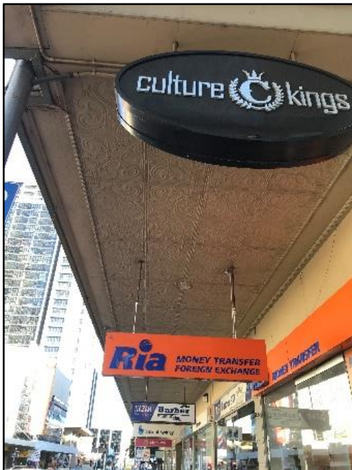
Figure 34. External view of the cantilevered awning showing the pressed metal ceiling of the Federation department store as viewed along Macquarie Street.
