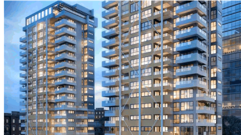
Imperial Towers complex could result in 179 apartments being added to housing supply once defects have been rectified and Practical Completion issued. Most of the 179 apartments have been pre-sold according to ABC News article 1 July 2021 ( https://www.abc.net.au/news/2021-07-01/nsw-parramatta-twin-towers-development-defects/100255704 )
