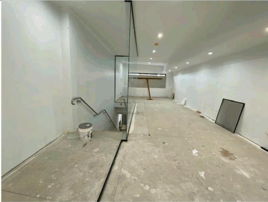
Figure 3: Office unit as built.
