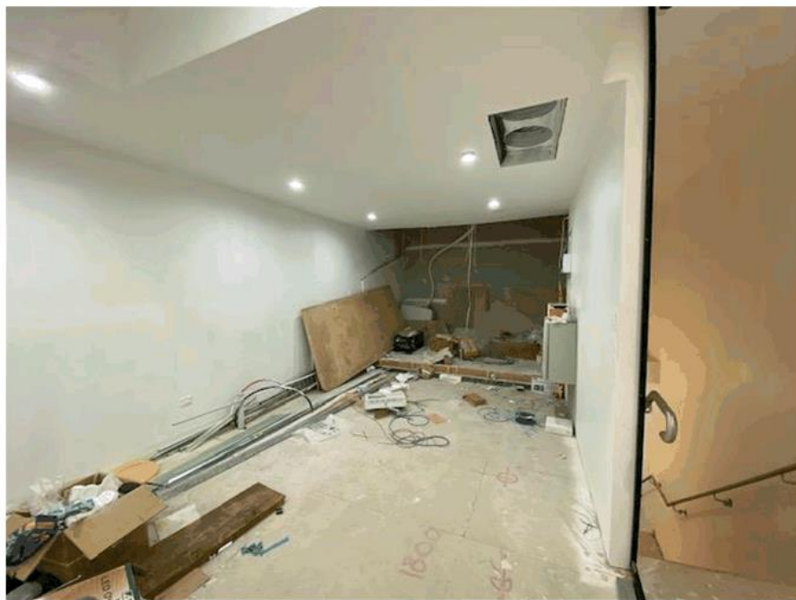
Figure 4: Office unit as built.
