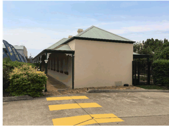
Figure 8 View of the western wing of the house, referred to as the barracks and the stables
