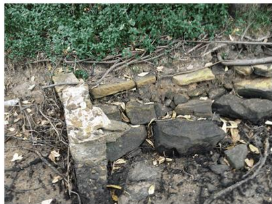
Figure 13 Potential remains of dock/ bathing area at the Parramatta River at the southeast corner of the site
