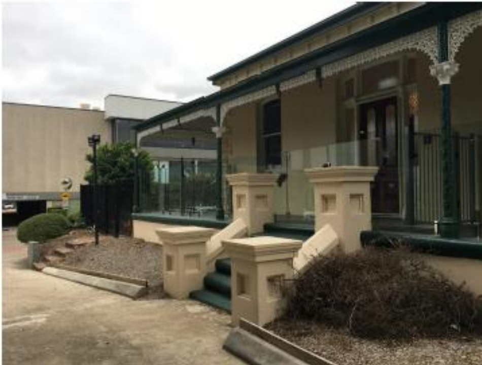
Figure 2: Truganini House (western frontage)
