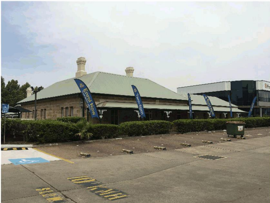
Figure 6 The northern and eastern facades of Truganini House
