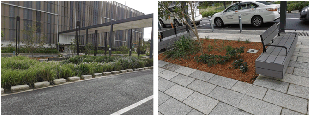
Figure 8.2.6.7.6.4 – WSUD at Northern Beaches Hospital
