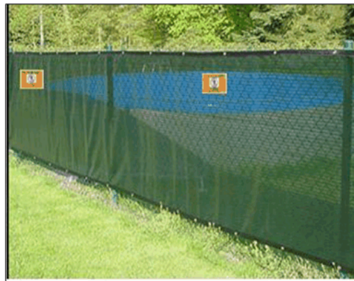
Figure 4: Tree Protection Fencing (collective)
