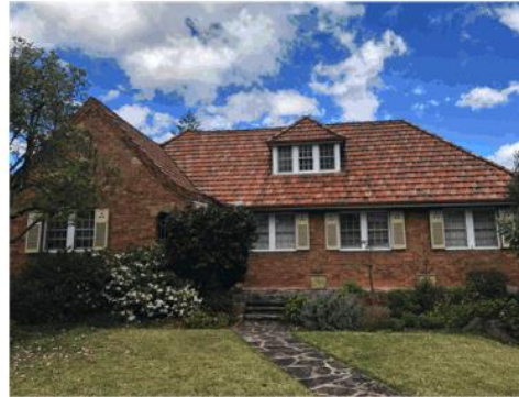
PHOTO 02 - FRONT OF EXISTING RESIDENCE FROM FRONT YARD
