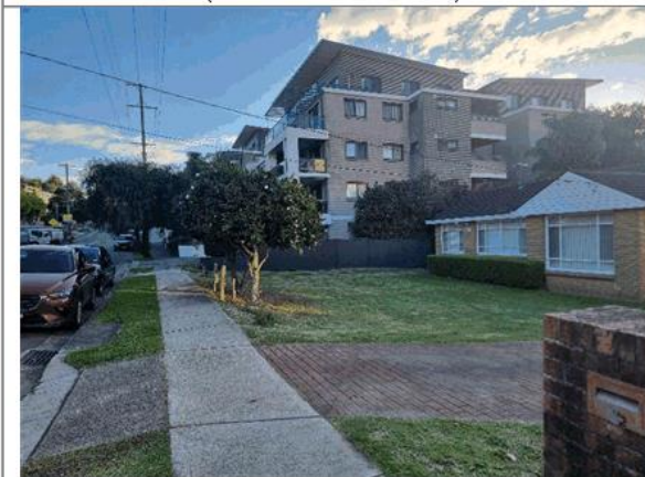
Figure 6: RFBs on Keeler Street further west of the site (Site Visit 20 June 2024)
