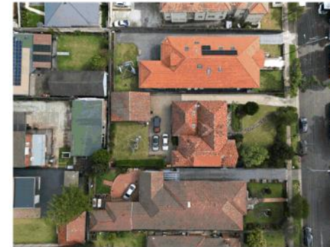
PHOTO 06 - AERIAL VIEW OF EXISTING RESIDENCE
