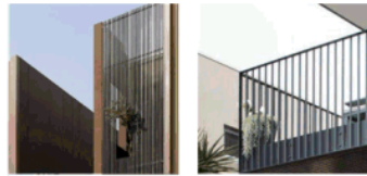
5. ALUMINUM LOUVRES WITH TIMBER LOOKING OR EQUIVALENT 6. VERTICAL BLADE ALUMINUM FENCE / BALUSTRADE WITH SIMILAR LOOK
