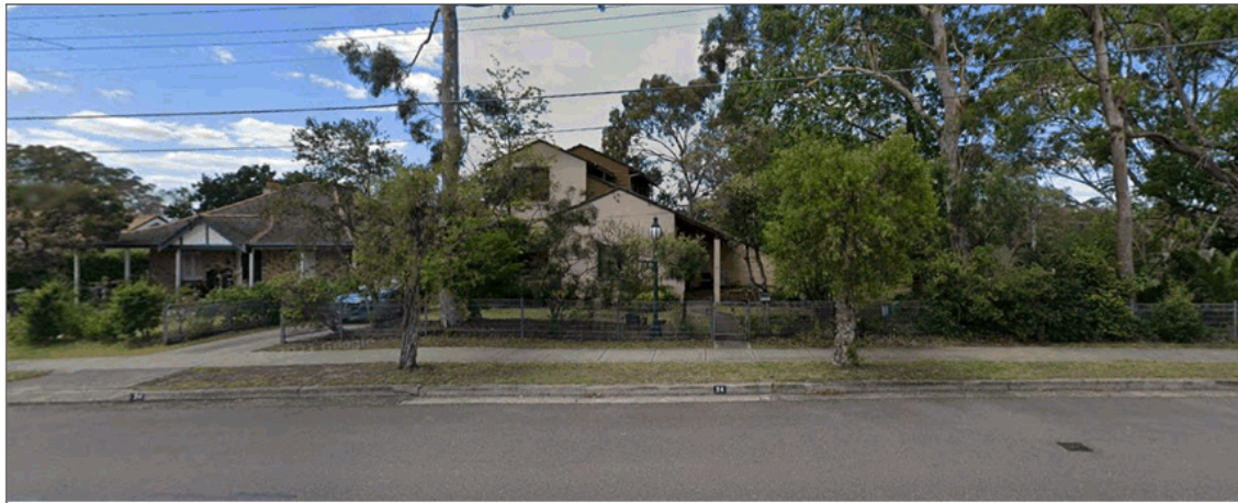
Figure 2: Subject Site, No. 24 Chesterfield Road, Epping
