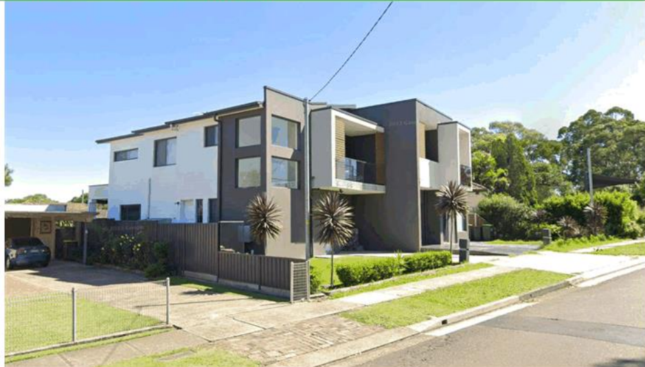
Photograph 3: Shows the recently constructed two storey attached dual occupancy on the opposite side of Crowgey Street.
