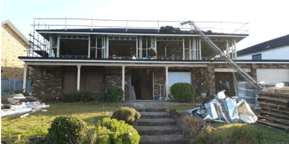
Figure 3: Subject site as viewed from Strathalbyn Drive. Source: Site Photo
