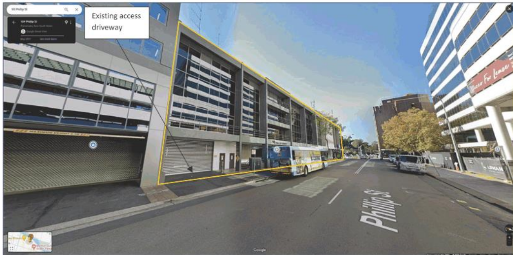
Figure 3 – Streetview image of the Phillip Street site frontage, looking east (Source: Google Maps)
