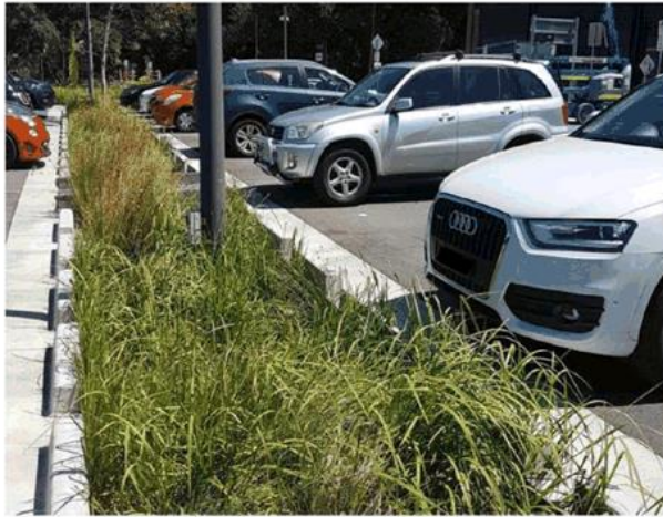
Figure 8.2.6.7.6.2 – Stormwater Swales (Source: Sydney Water – ‘Water Sensitive Urban Design’ SW277 03/18)
