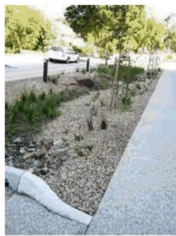
Figure 8.2.6.7.6.2 – Stormwater Swales (Source: Sydney Water – ‘Water Sensitive Urban Design’ SW277 03/18)
