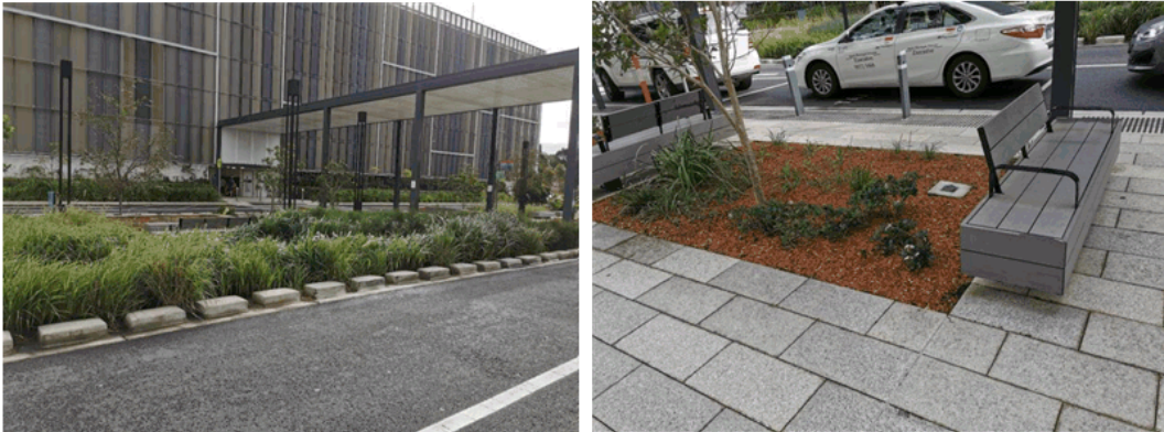
Figure 8.2.6.7.6.4 – WSUD at Northern Beaches Hospital
