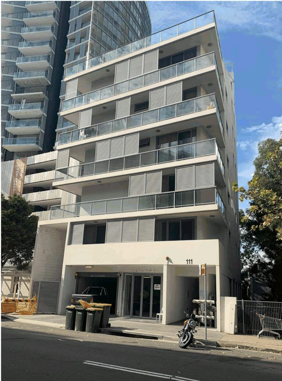
Photograph 5: Mixed Use Development located at No. 111 Wigram Street, Harris Park
