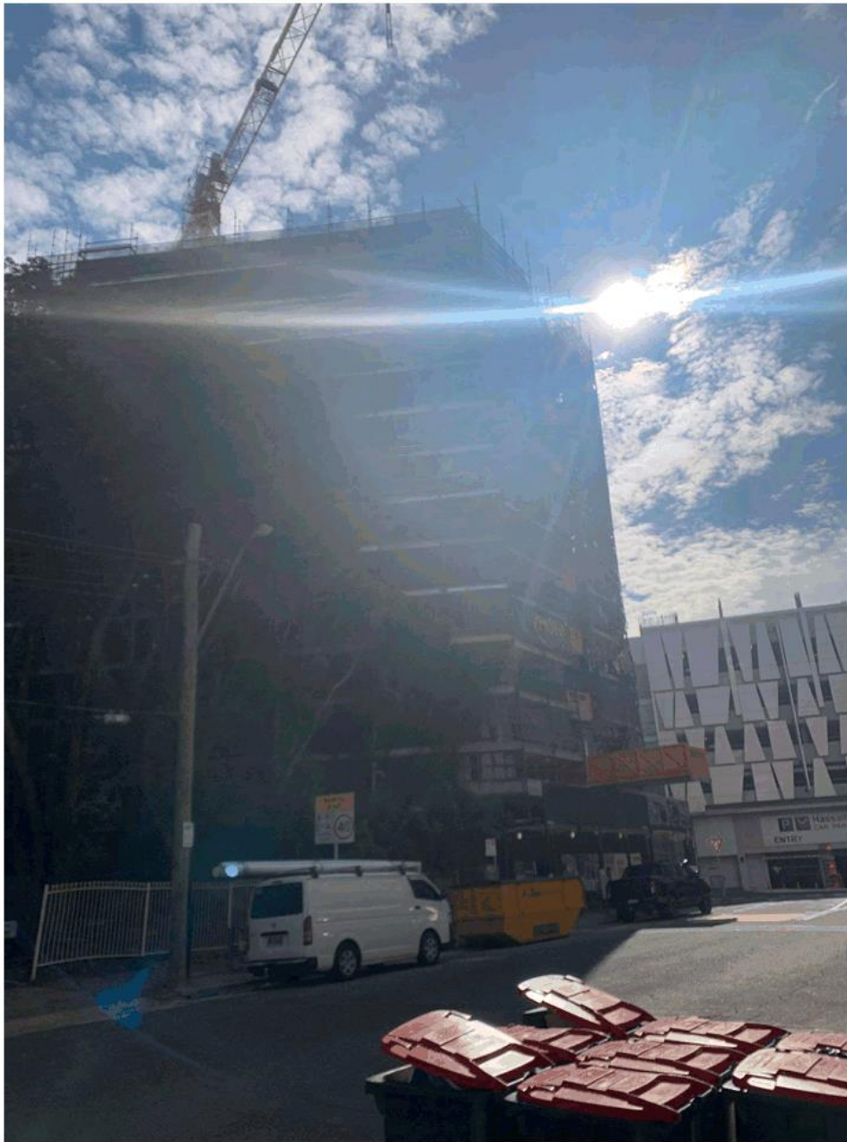
Photograph 6: Earlier construction taking place to the site (No. 21 Hassell St)
