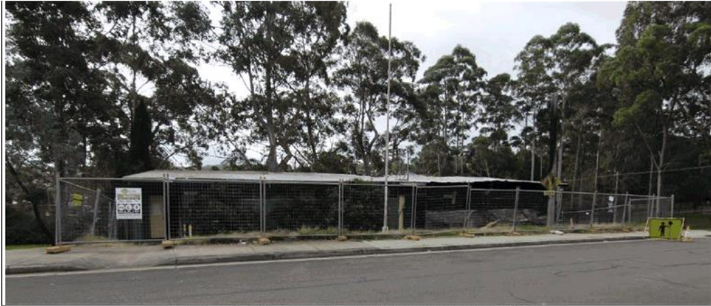
Figure 3. Front elevation of scout hall viewed from Fullford Street
