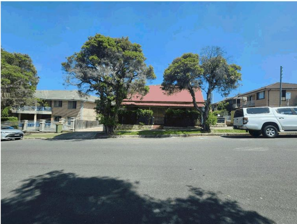
Figure 7: View of site as seen from Isabella Street (Site inspection, 29/01/2024).
