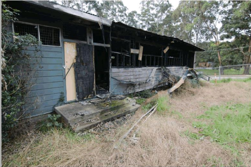
Figure 4. Front elevation of scout hall viewed from Fullford Street.
