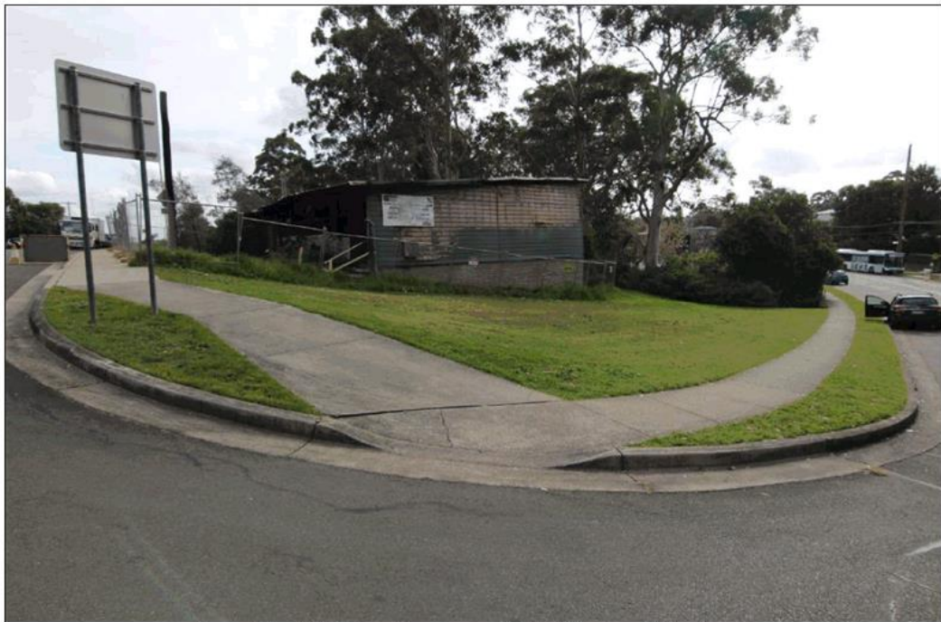
Figure 4. Scout hall viewed from corner of Fullford Street and Yates Avenue.
