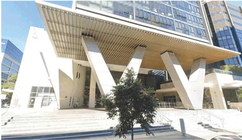
Figure 9 – Street view of the subject site from Macquarie Street, Parramatta
