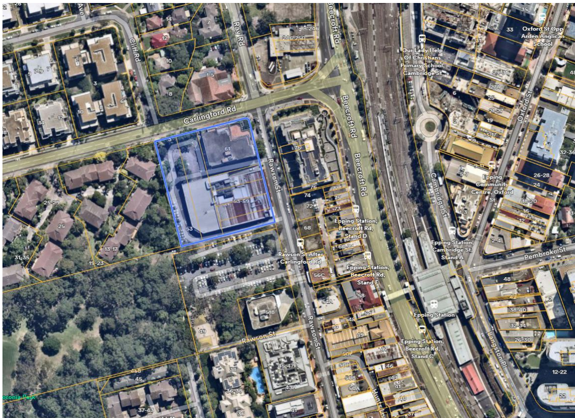
Figure 1: Subject site at 53-61 Rawson Street, Epping (source: NearMap)
