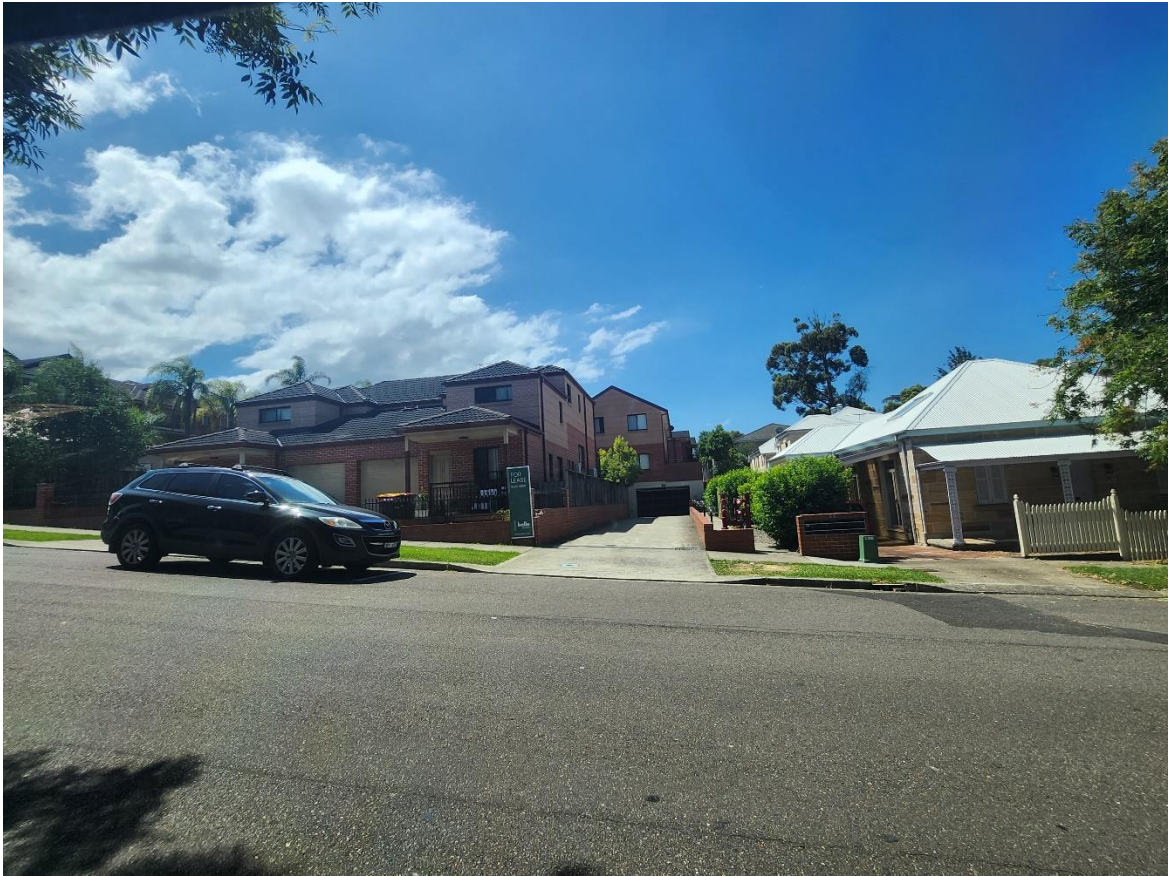
Figure 6: View of site looking directly north from Albert Street (Site inspection, 29/01/2024).
