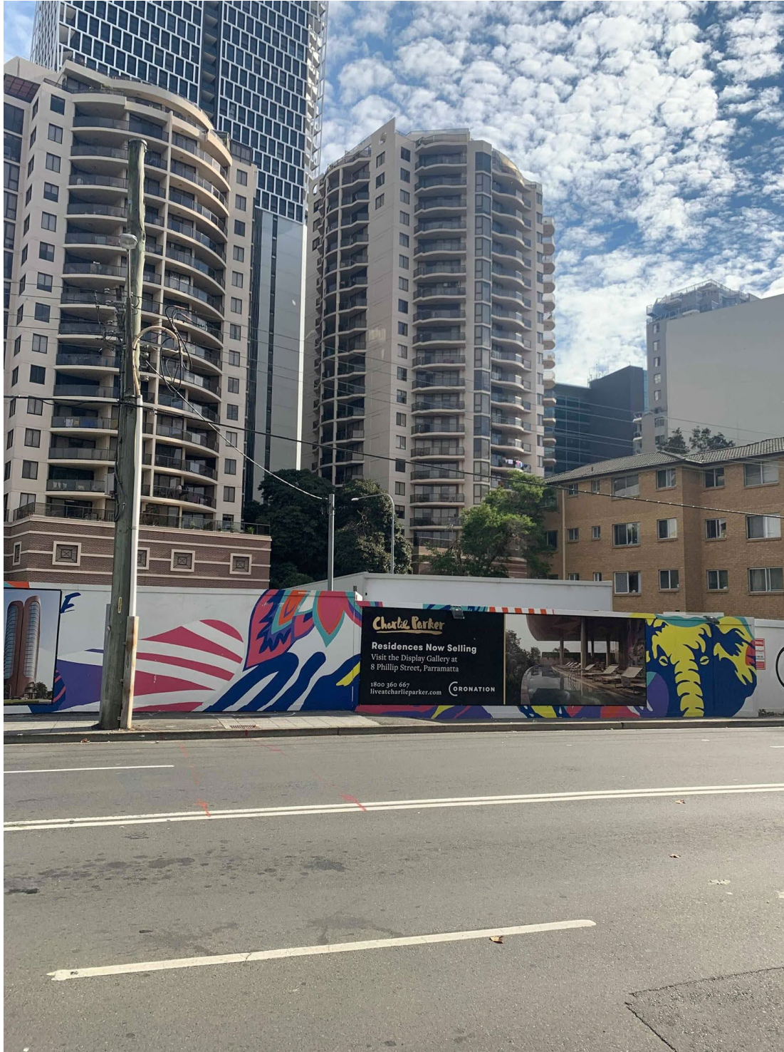
Photograph 4: Shows the adjoining site 12A Parkes Street, Harris Park
