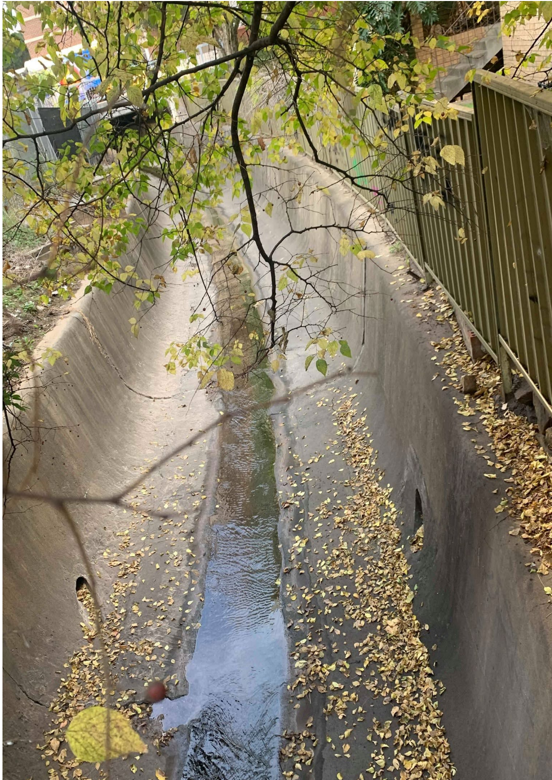
Photograph 3: Shows the concrete channel that runs along the southern site boundary
