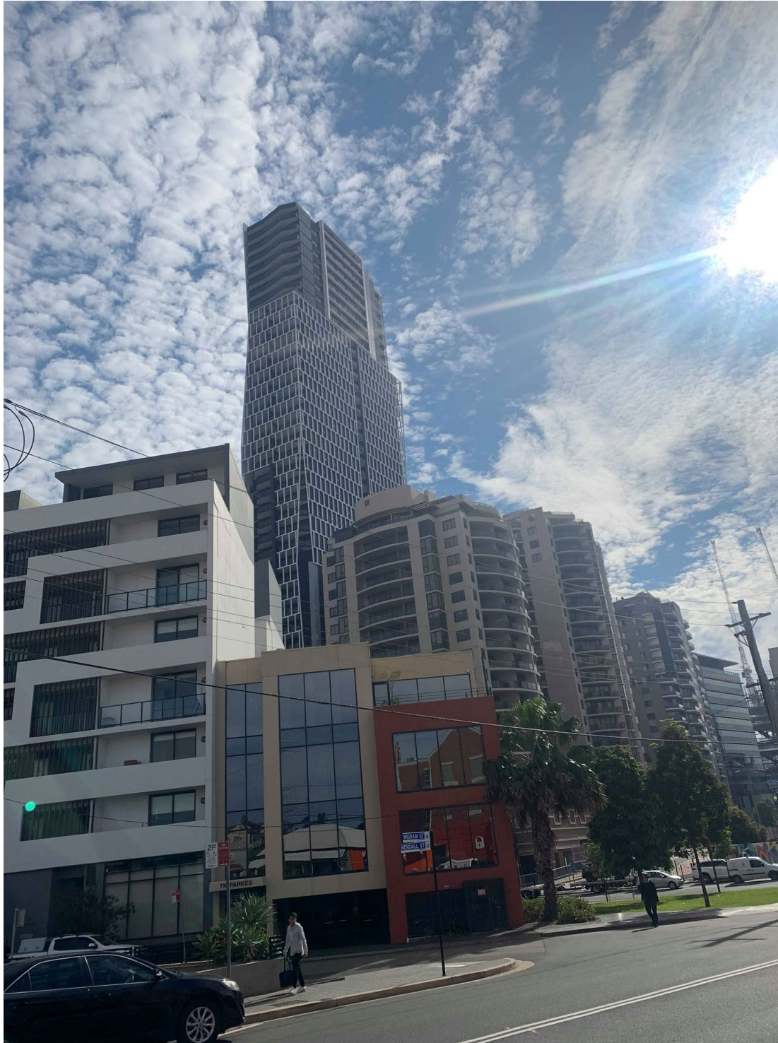
Photograph 2: Shows the built form pattern as viewed from Wigram Street
