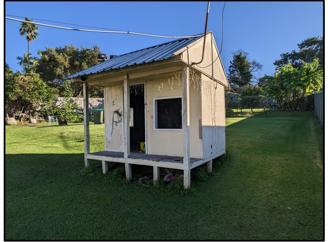
Figure 12. Fibrocement building within eastern portion of the site.
