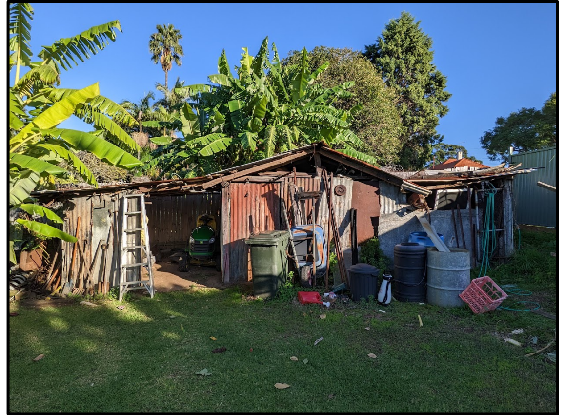
Figure 14. Metal shed within north-western portion of the site.
