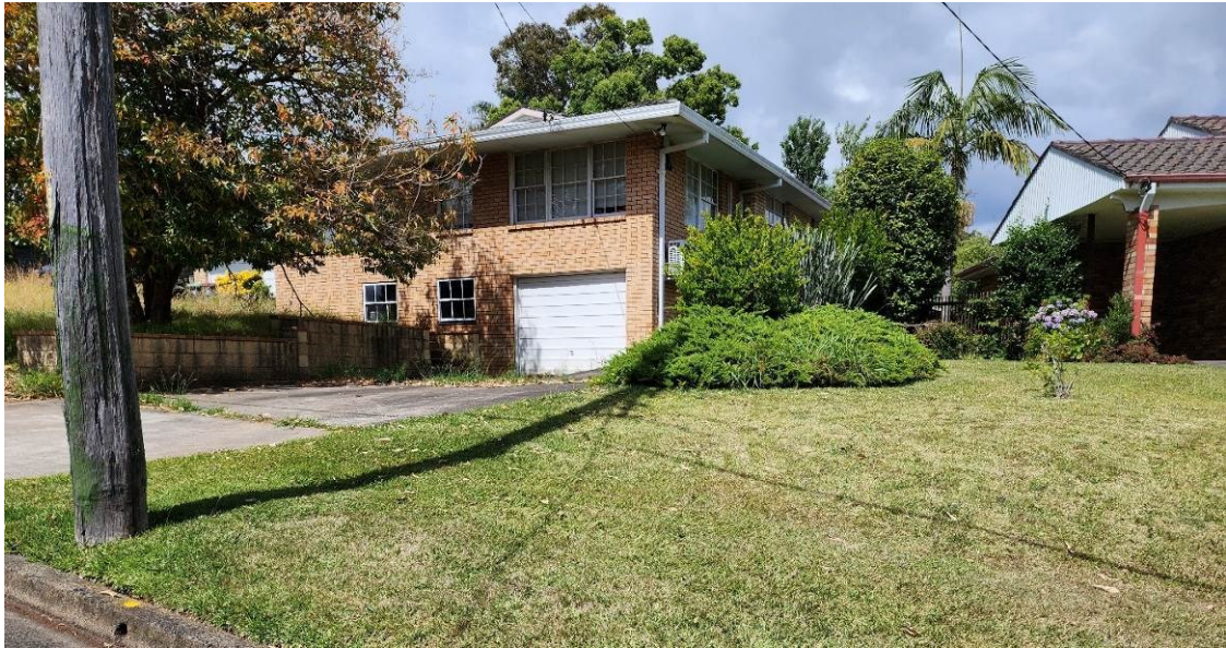
Figure 8: Photograph of No. 3 Tracey Avenue
