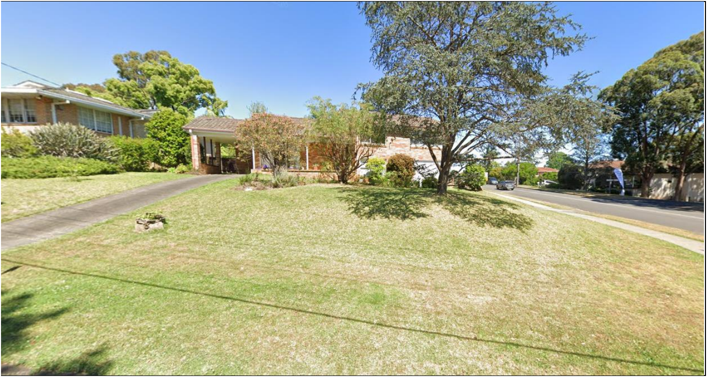
Figure 3: Subject site viewed from 1 Tracey Avenue. (Site inspection, 11 October 2023)
