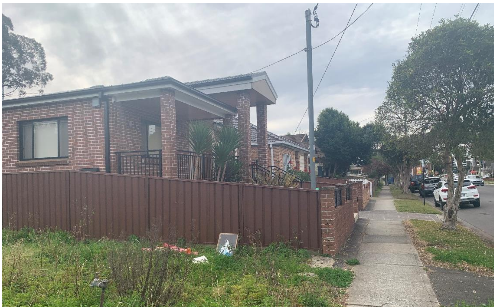
Figure 4: Adjoining site to the north (142 Alfred Street) as viewed from Alfred Street. Source: Site Inspection.
