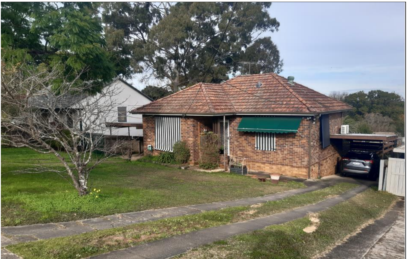
Figure 4: Subject site (8 Manson Street). Source: Site Inspection (29/06/22).
