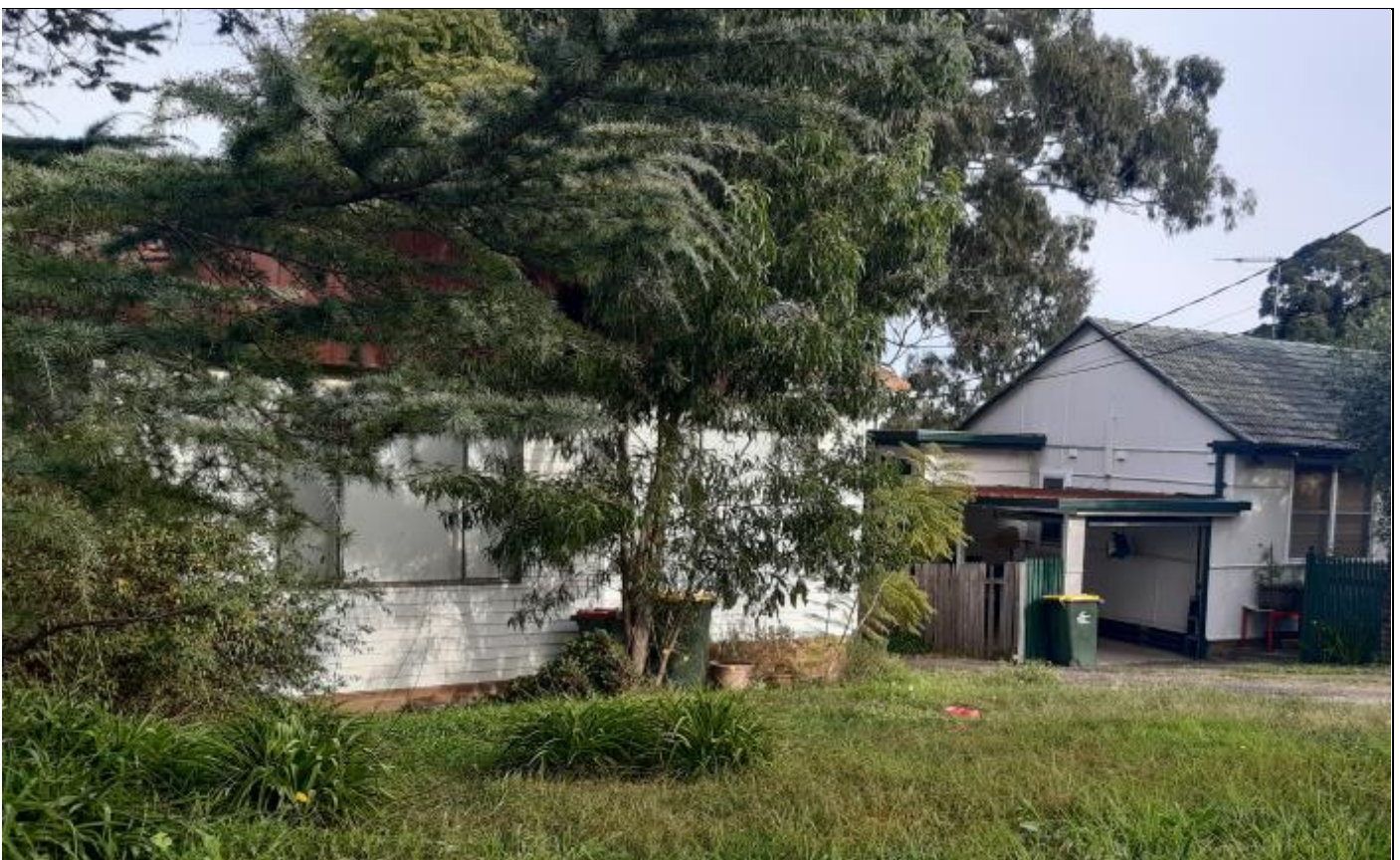
Figure 6: Subject site (12 Manson Street). Source: Site Inspection (29/06/22).
