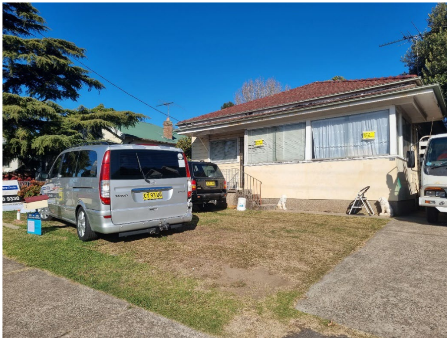
Figure 2: Subject site from Victoria Road. Source: Site Inspection.
