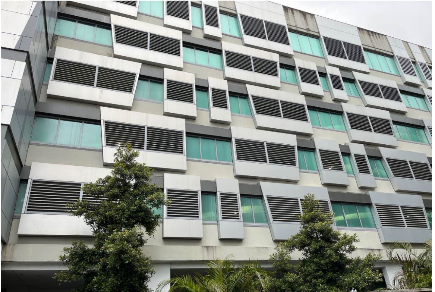
Figure 8 - Photo of adjoining above ground carpark at 189 Macquarie St (Source: Think Planners, 2022)
