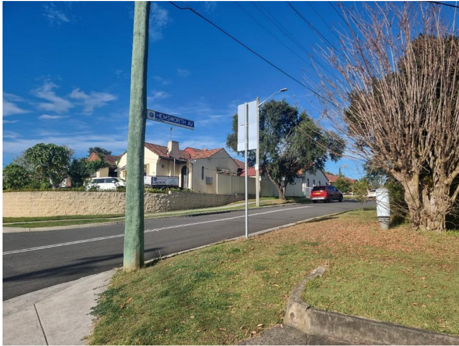
Figure 4: View of developments opposite the subject site on Hemsworth Avenue. Source: Site Inspection
