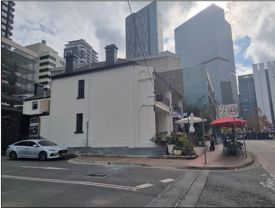
Figure 5: Existing Heritage Item located across Woodhouse Lane looking north
