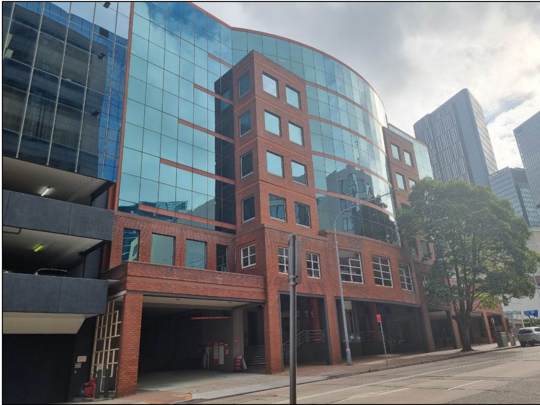
Figure 2: Subject site as viewed from Wentworth Street looking north-west
