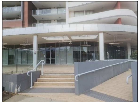
Figure 6: Subject Site looking south from river walkway.
