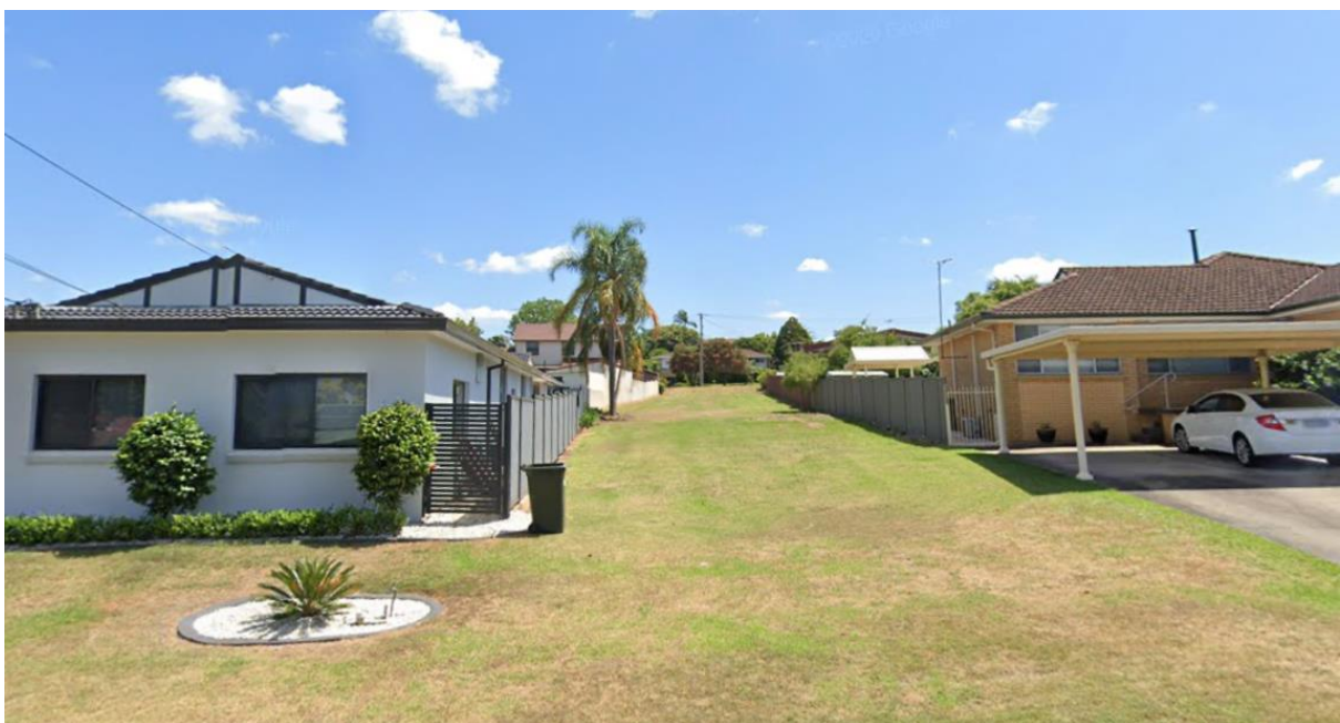
Figure 7 – Neighbouring site at 10 and 10A Lloyd George Avenue (Google Maps, 2022)
