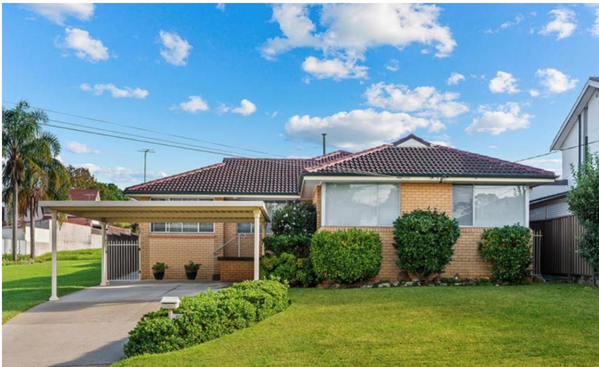
Figure 3 – Subject site as viewed from Lloyd George Avenue (Realestate.com.au, 2022)
