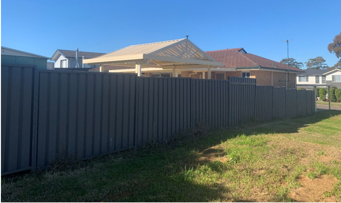
Figure 7: 12 Lloyd George Avenue, Winston Hills from the adjoining public reserve facing south east. Source: Site inspection
