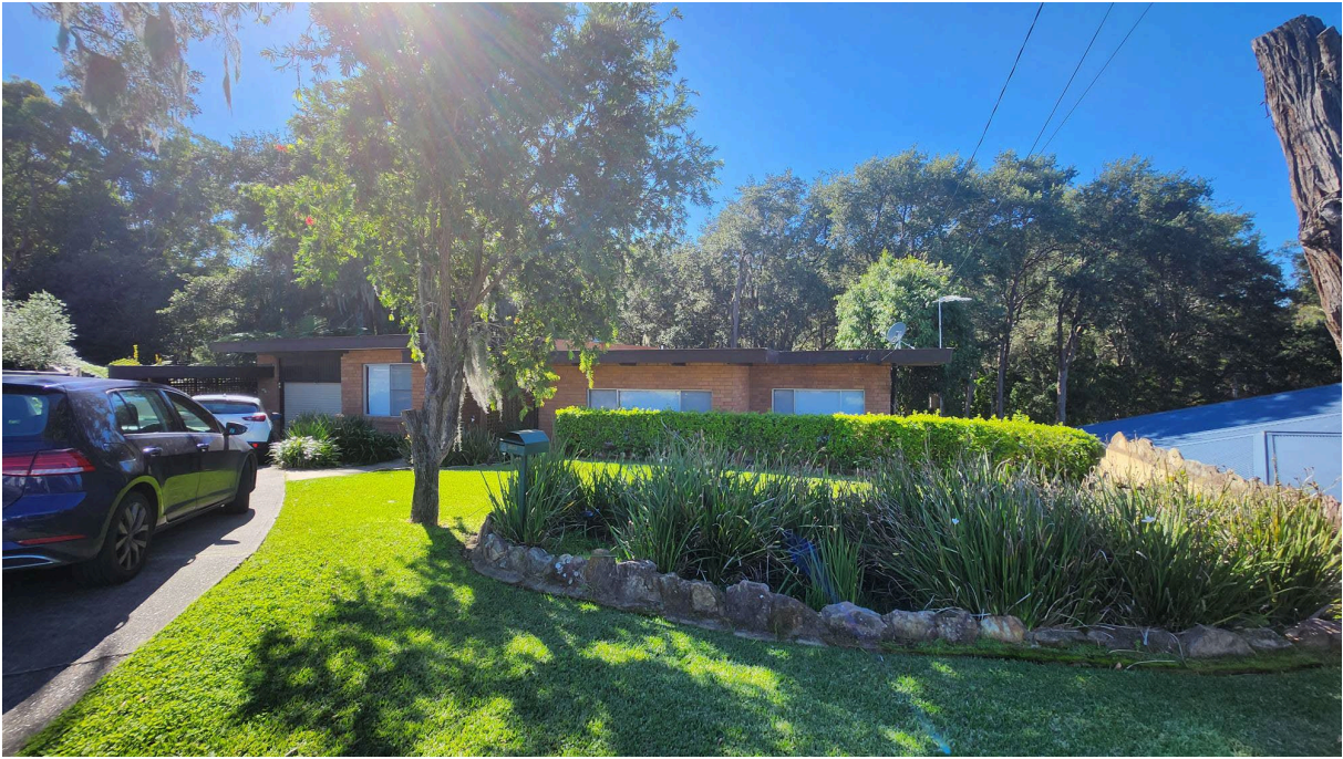
Figure 5: View of site as seen from Stringer Place (Site inspection, 10 May 2023).
