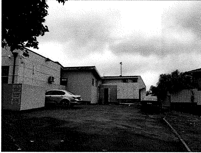
Area of proposed development - Looking south to the loading dock area
