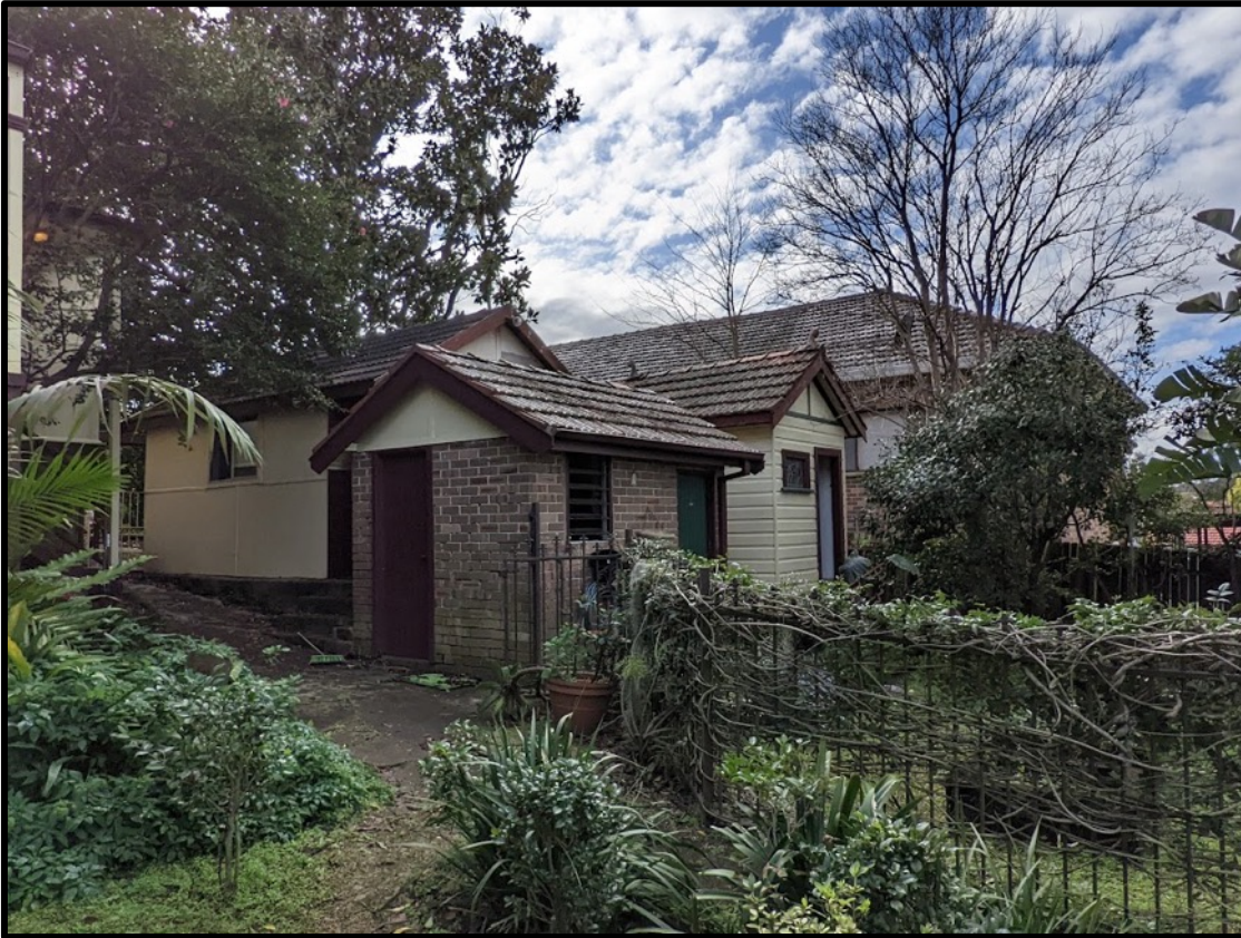
Figure 9. rear view of the garage shed, brick and weatherboard shed within the eastern portion of the site.
