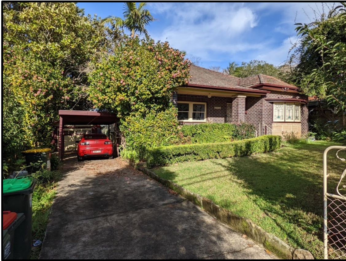
Figure 7. Front view of the brick dwelling, lawn area and concrete driveway.
