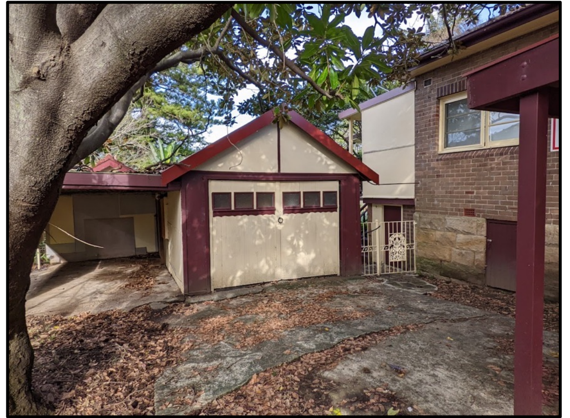
Figure 8. Garage fibrocement shed and canopy within the eastern portion of the site.
