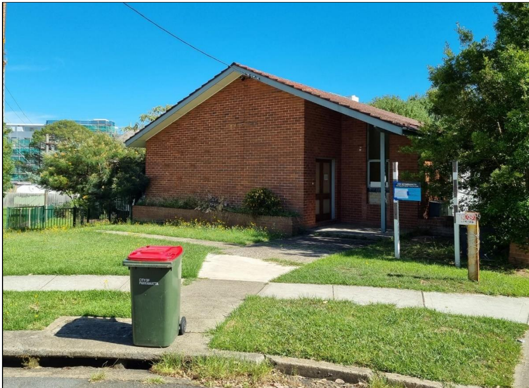
Figure 1: Subject site as viewed from St Andrews Street. Source: Site Inspection.
