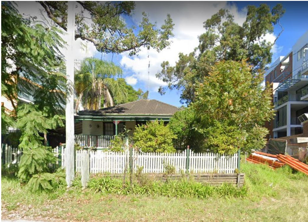
Figure 2: Subject site as viewed from Kissing Point Road. Source: GoogleMaps.
