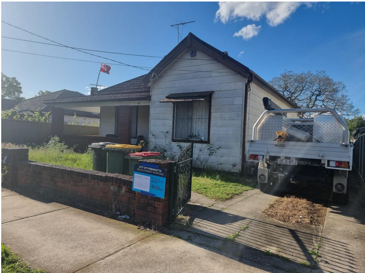
Figure 2: Subject site as viewed from Boundary Street. Source: Site Inspection.
