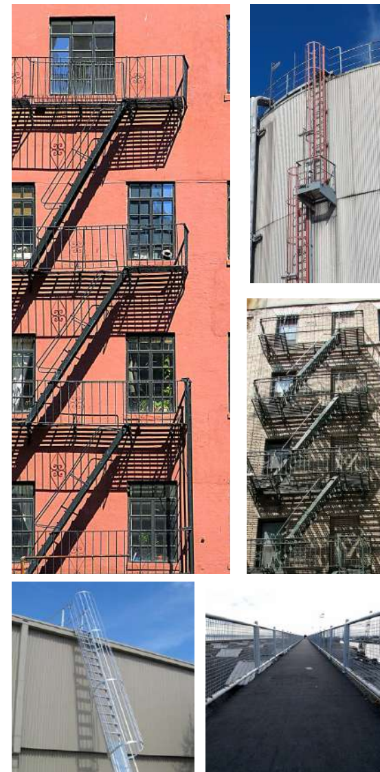
Examples of lightweight high level access/escape solutions.
