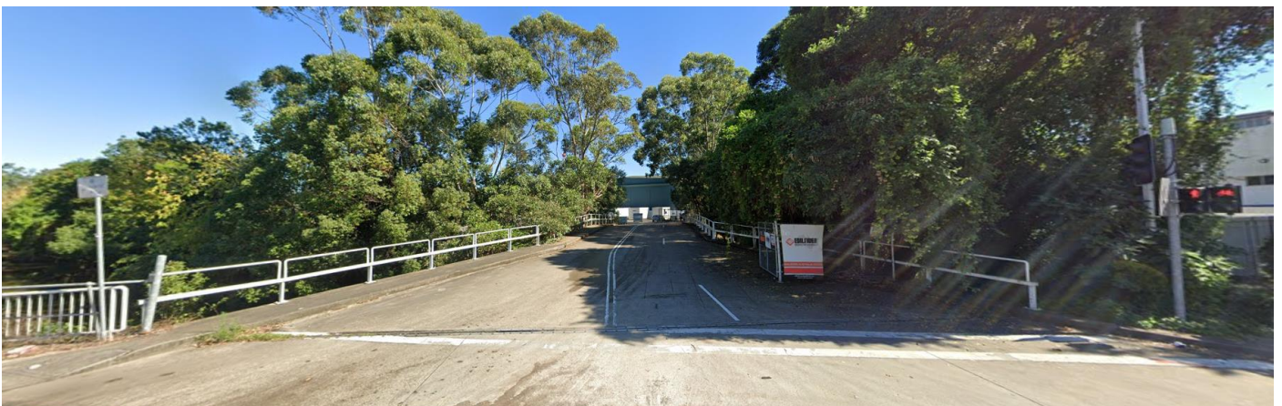
Figure 2: Existing elevated concrete bridge connecting the subject site to North Rocks Road
