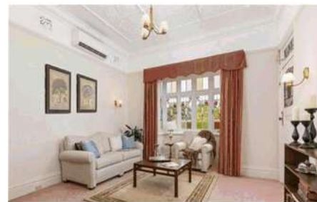
Figures 10 and 11: The front bedroom and sitting room of No 16 Victoria St, Epping feature typical Federation Bungalow elements such as high ceilings with decorative plasterwork and ceiling roses, high skirtings, ornate architraves and leadlight panels in casement windows. Source: Realestate.com.au 2020
