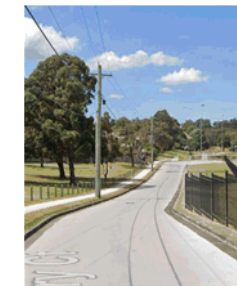
7. REMOVE SECURITY FENCING & BOLLARD POSTS
