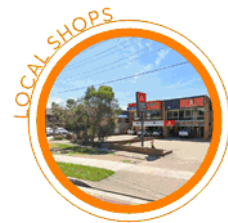
Shopping Facilities, Victoria Road
